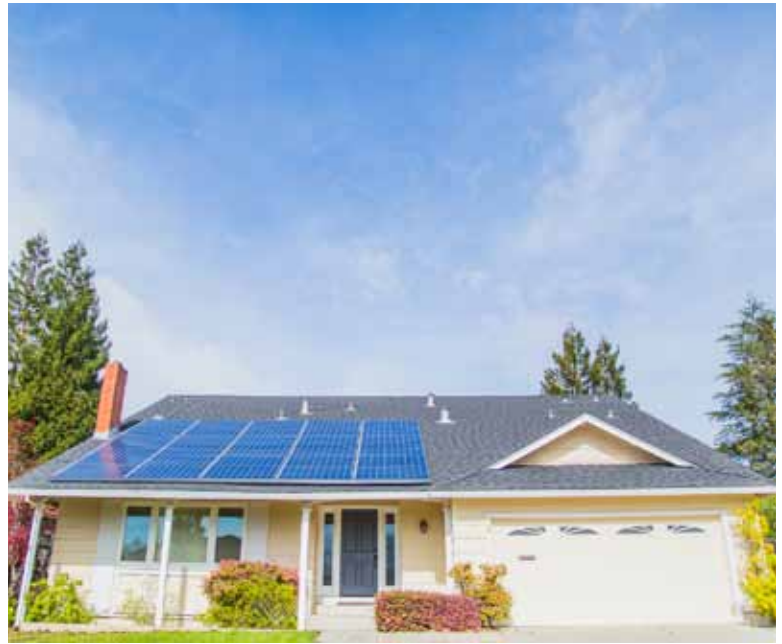
Increasing numbers of solar panels installed on residential rooftops, like the one pictured above, are helping to reduce dependence on fossil fuels. (Photo: SolarCity)
